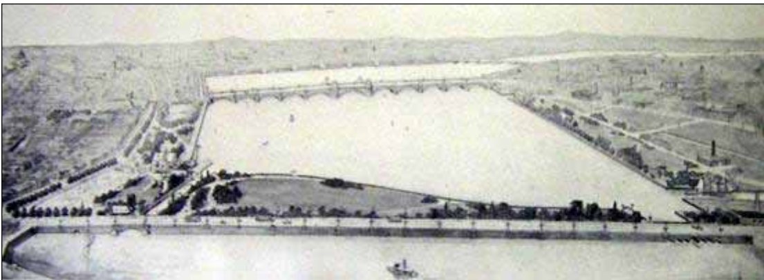
Figure 2.3 – 1904 aerial perspective showing proposed Charles River Dam in the foreground, Longfellow Bridge in the background and Charlesbank at far left with gatehouse and pump house on newly filled land adjacent to the lock. (DCR Archives)
