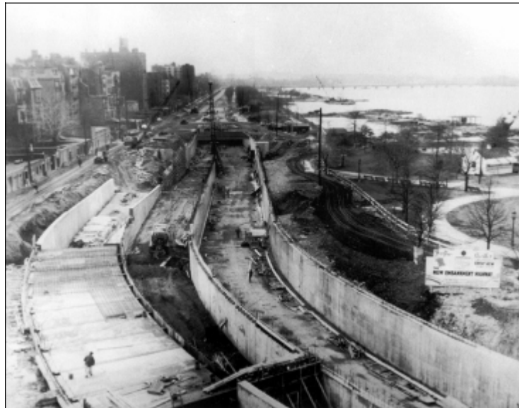
Figure 4.1 – This 1951 view shows construction of the Storrow Drive Tunnel with fill from the tunnel used to create additional parkland. (from Mapping Boston)
