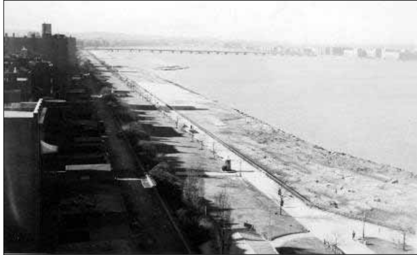
Figure 3.11 – Aerial view of Back Bay section under construction in 1933. The wide central path marks the former edge of the Esplanade. The land to the right of it is new fill. The lagoon is in the background in this photo and the one below. (DCR Archives)
